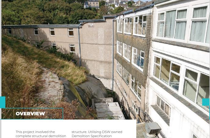
This project involved the complete structural demolition of a former hotel. Compliant licensed and non-licensed ACM removal was undertaken by a sub-contractor.
